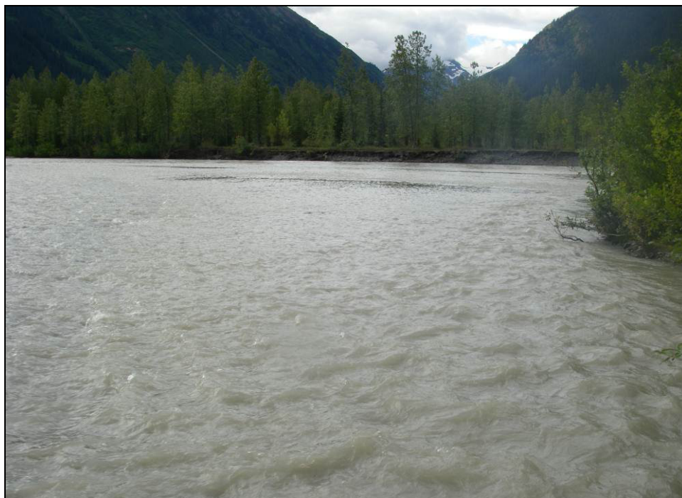
Plate 7.2-2. A view of the Bowser River at Site 1 with little cover and eroding banks.
