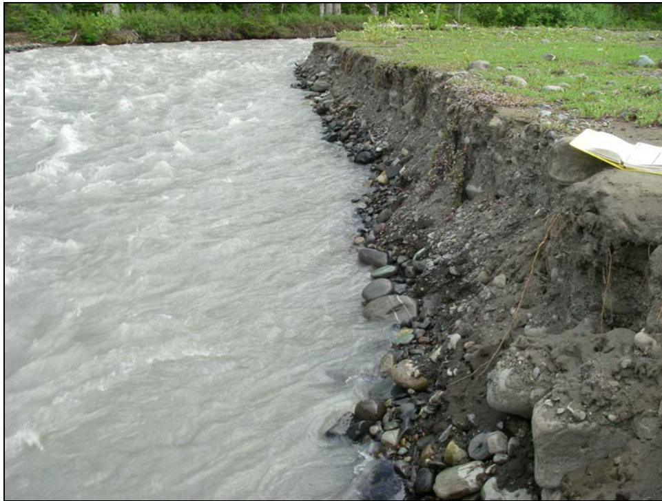
Site # 108 Photo: IMG3966 Site 108 - The banks at the bottom end of the site showed evidence of erosion.
