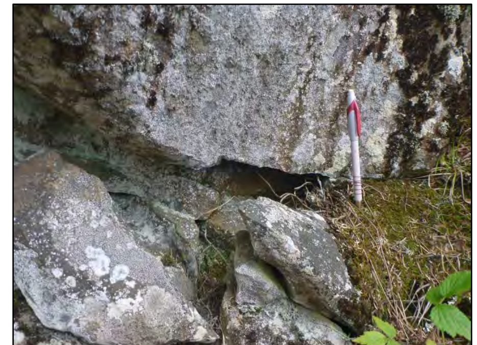
Photo 12: Crevice observed at 115lo
