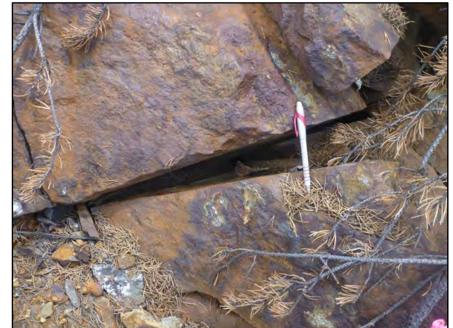
Photo 17: Crevice observed at 100med
