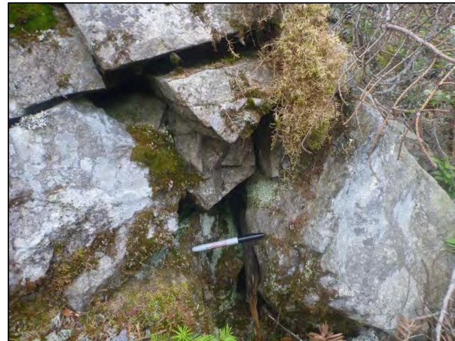
Photo 15: Crevice observed at 117lo
