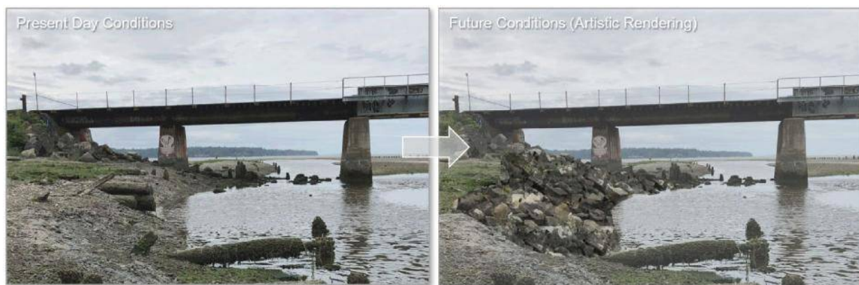
Figure 4.6 (Left) Present day conditions at the project site. (Right) Artistic rendering of Opportunity 5 – East River Bank Protection. Note that the rendering is indicative only.
