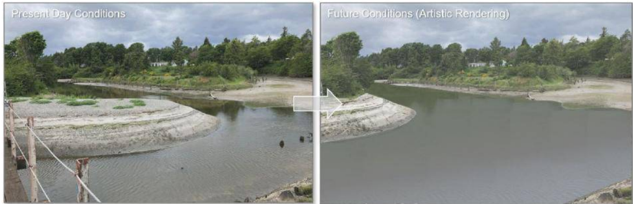
Figure 4.7 (Left) Present day conditions at the project site. (Right) Artistic rendering of Opportunity 6 – Sediment Lobe Removal. Note that the rendering is indicative only.
