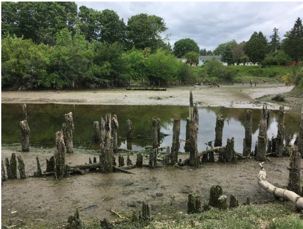
Figure 8: Northeast View of Remnant Piles Proposed to be Removed as part of the Semiahmoo Project (Taken May 22, 2020)
