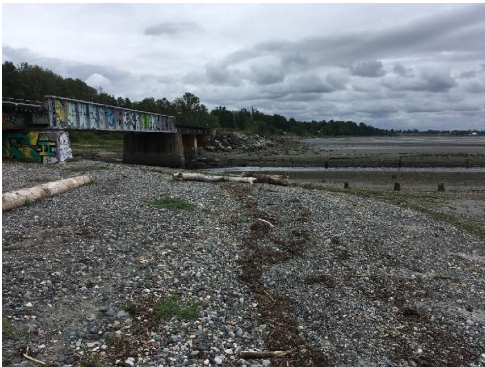
Figure 12: East View of Western Semiahmoo Bay Foreshore Area Targeted for Groyne Implementation and Sandy Gravel Beach Enhancement as part of the Semiahmoo Project (Taken May 22, 2020)
