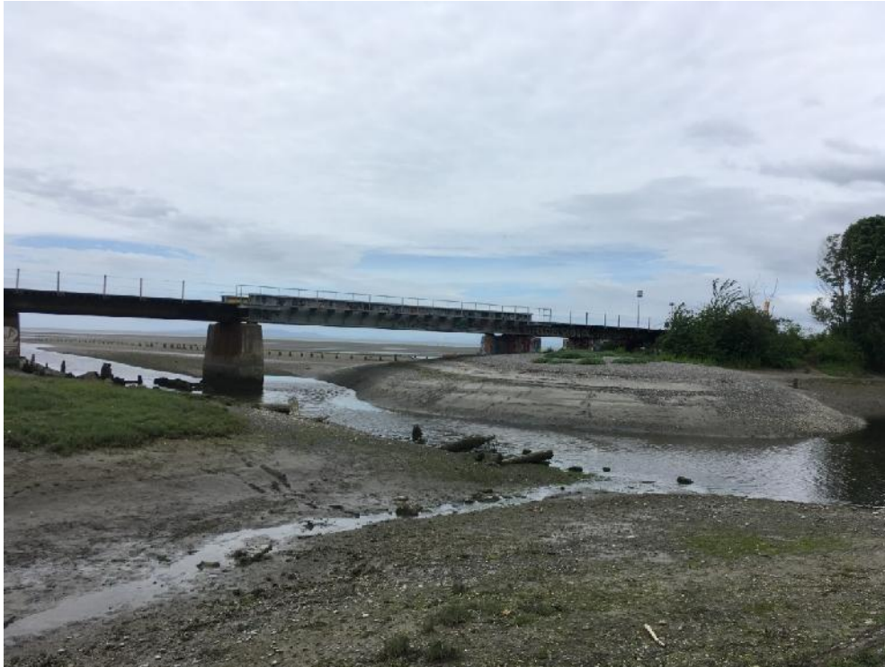
Figure 11: Southwest View of the Little Campbell River Mouth and the East and West Bank Areas Proposed for Armouring and Sediment Removal as part of the Semiahmoo Project (Taken May 22, 2020)
