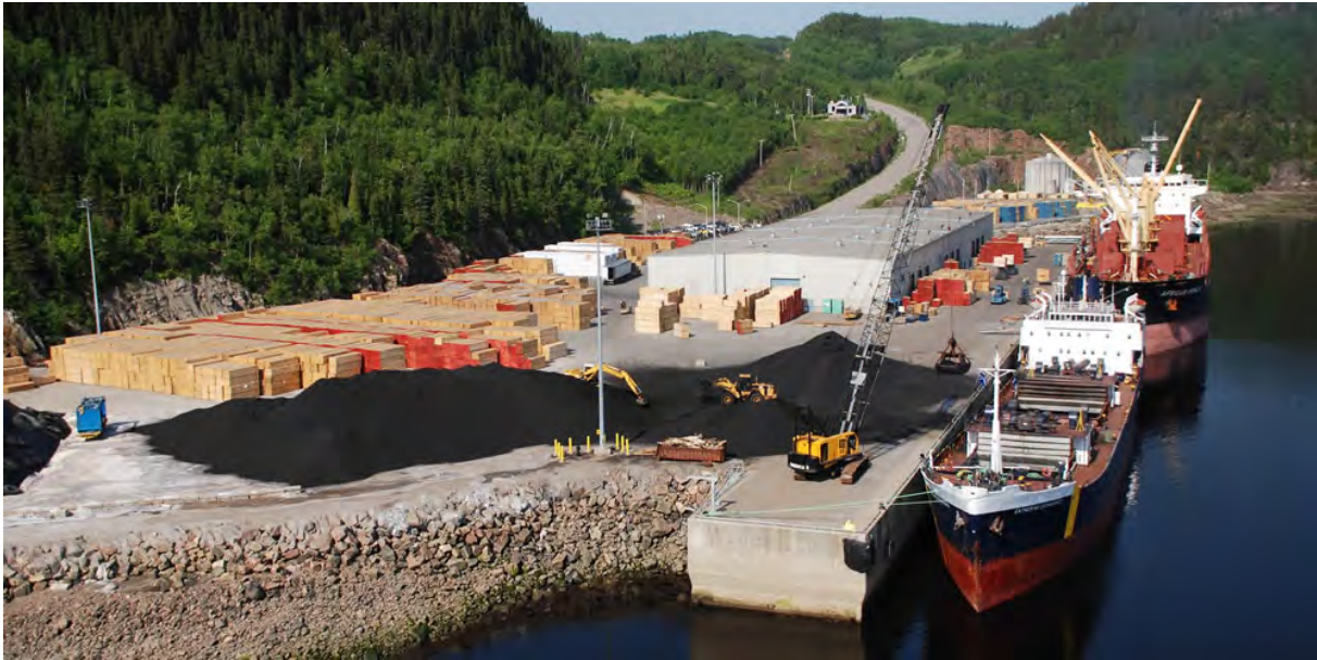
Figure 3. Grande-Anse Marine Terminal.
