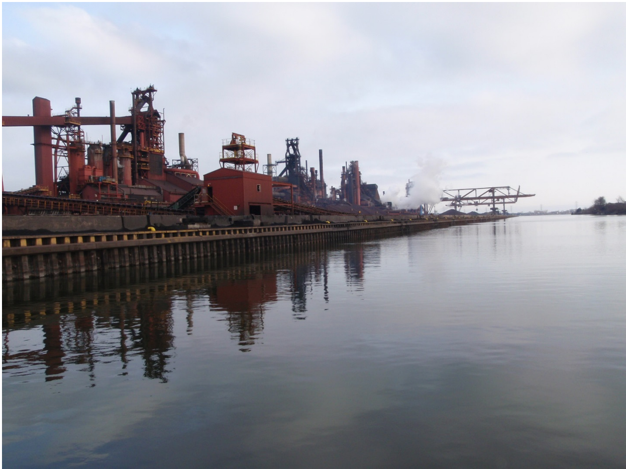
Photo 3 View of ArcelorMittal Dofasco Boat Slip
