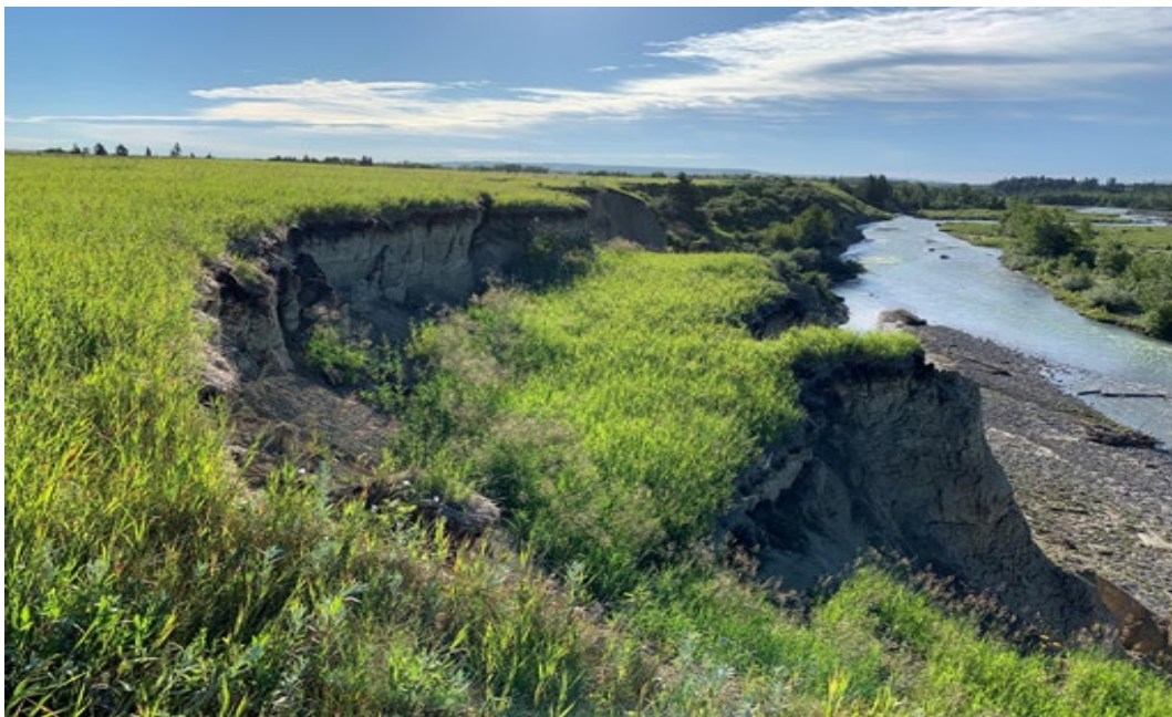
Photo 5 Bank Swallow Colony Location and Slope Failure along Elbow River (BANS_BY02)
