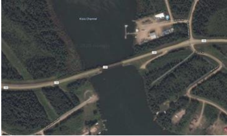
Water Feature No 19 – Kisis Channel & Bridge
