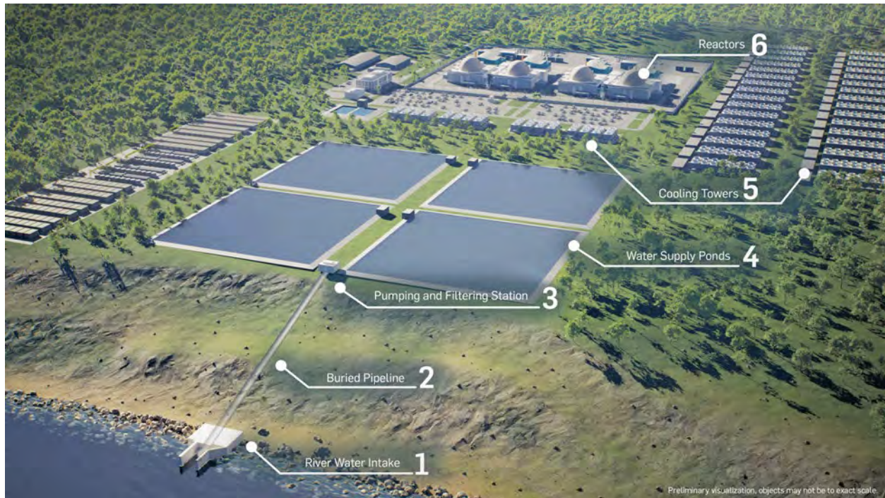
Figure 4.4-3: Site Cooling Water Infrastructure Diagram
